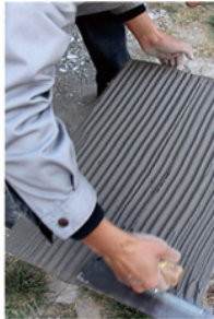
2 Make mortar into stripe pattern
