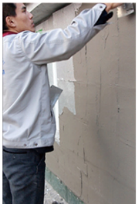
5 Coat Vokes®HVIP with mortar
