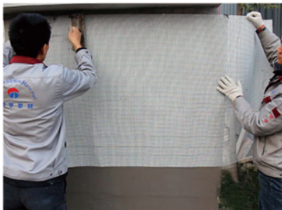
6 Paste mesh fiber on mortar
