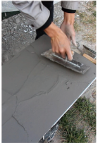
1 Apply adhesive mortar on Vokes®HVIP
